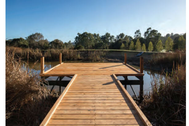
TIMBER BOARDWALK AND DECK TO DRAINAGE BASIN
